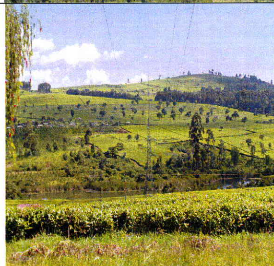
View of existing line in Nandi Hills area
