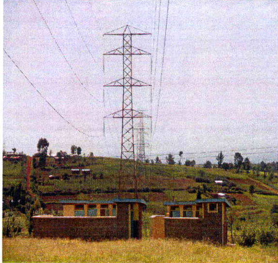
Toilets at Jogoo Primary School, Molo – built under existing transmission line
