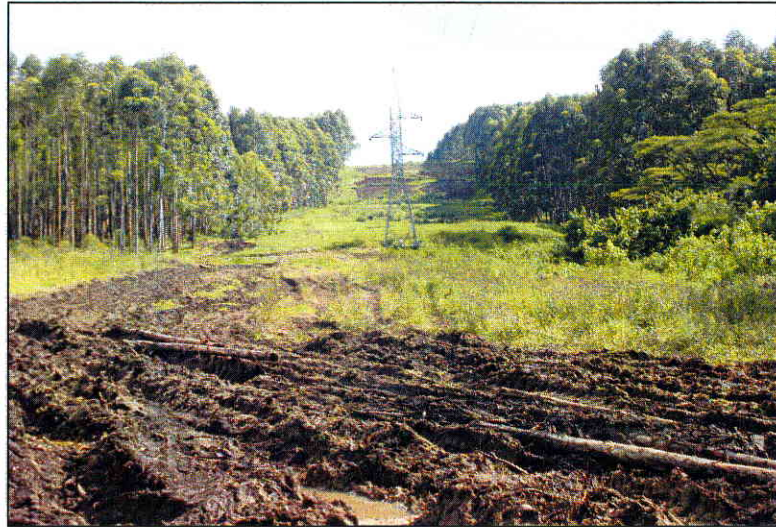
Fig 7-10: Visual impact of transmission line and towers on forest land – Nandi Hills
