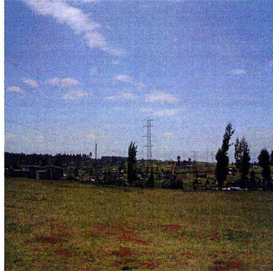
View of structures likely to be lost/ affected on the right-hand-side of the existing transmission line, taken at Mau Summit Area, Koige Village
