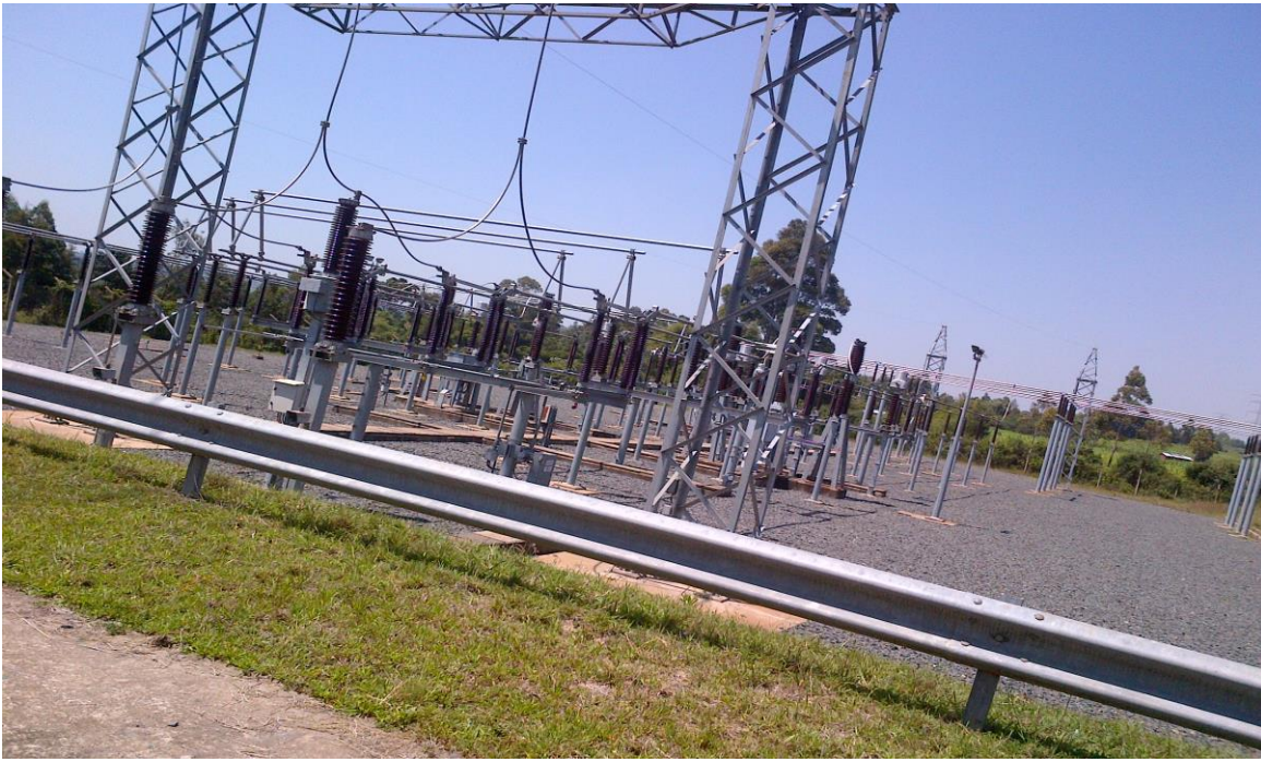
Plate 3: Existing substation to be expanded
