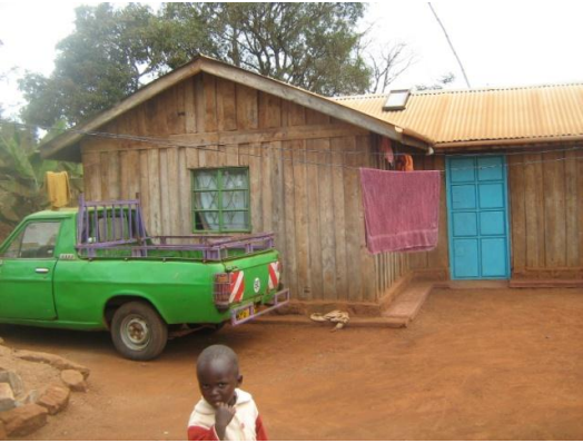
A view of structure at Mbeti North Location near proposed substation proposed for relocation
