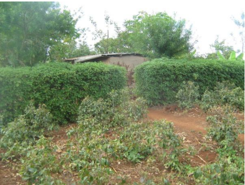
A view of a structure at AP 8 proposed for relocation
