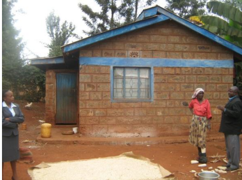
A view of structure at Kithimu Location proposed for relocation
