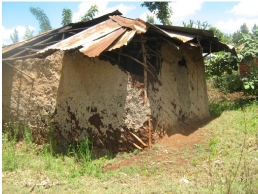
A view of a structure at AP7 proposed for relocation
