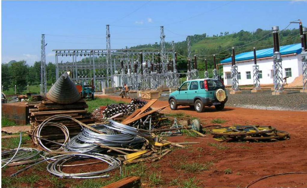
Typical materials and waste in construction of power lines
