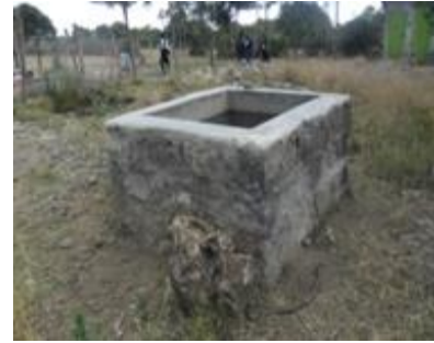
Water open tank
