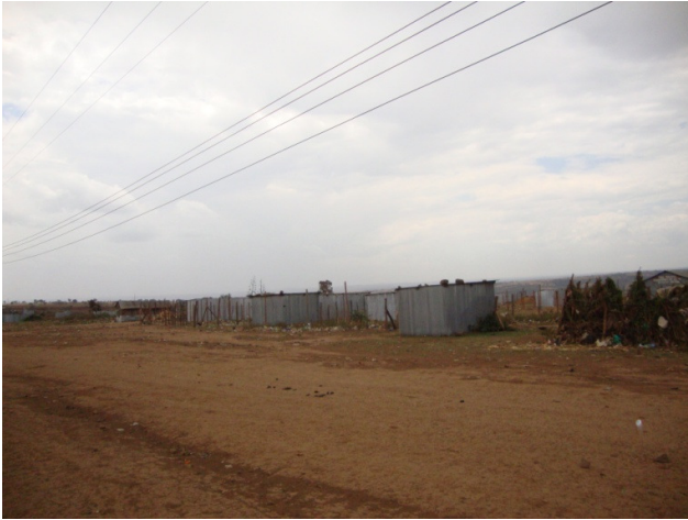
Fig. 3.8: Temporary structures neighbouring the existing 33kV line at Ntulele Centre
