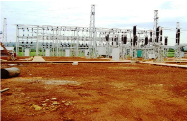
Fig.3.10: Kegati Substation under construction
